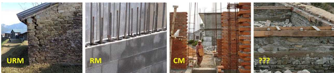
Fig. 4 - Three existing masonry categories: Unreinforced (URM), Reinforced (RM), Confined (CM), and a newly proposed 4 th category of Nominally Reinforced Masonry (NRM).
